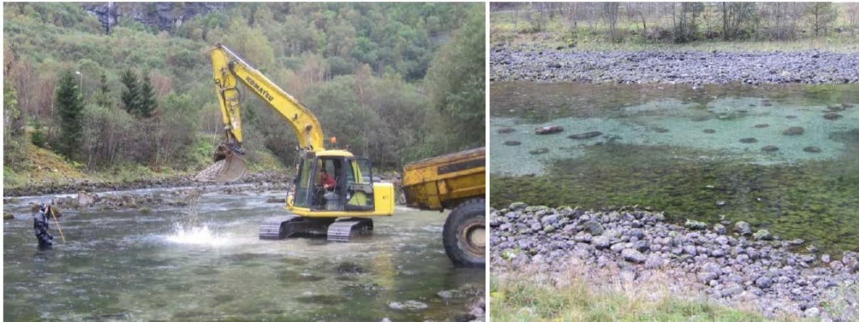
Figure 4-2. Placement of spawning gravel in Aurlandselvi in Norway, under the supervision of a researcher (from Pulg et al. 2007).
