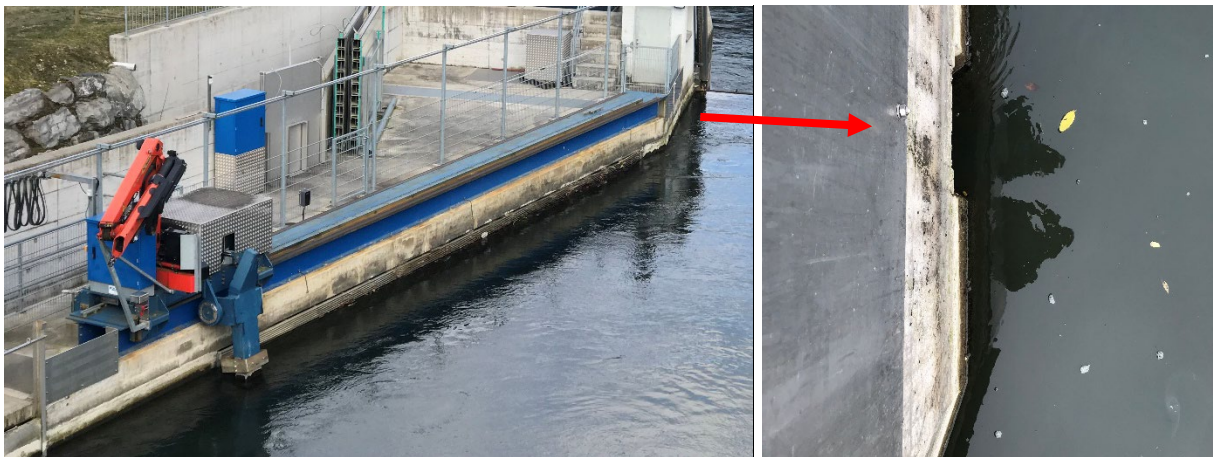
Figure 5: Plan view illustration (top), photo (middle) of HPP Schiffmühle and close-up photo of HBR & bypass inlet (bottom).
