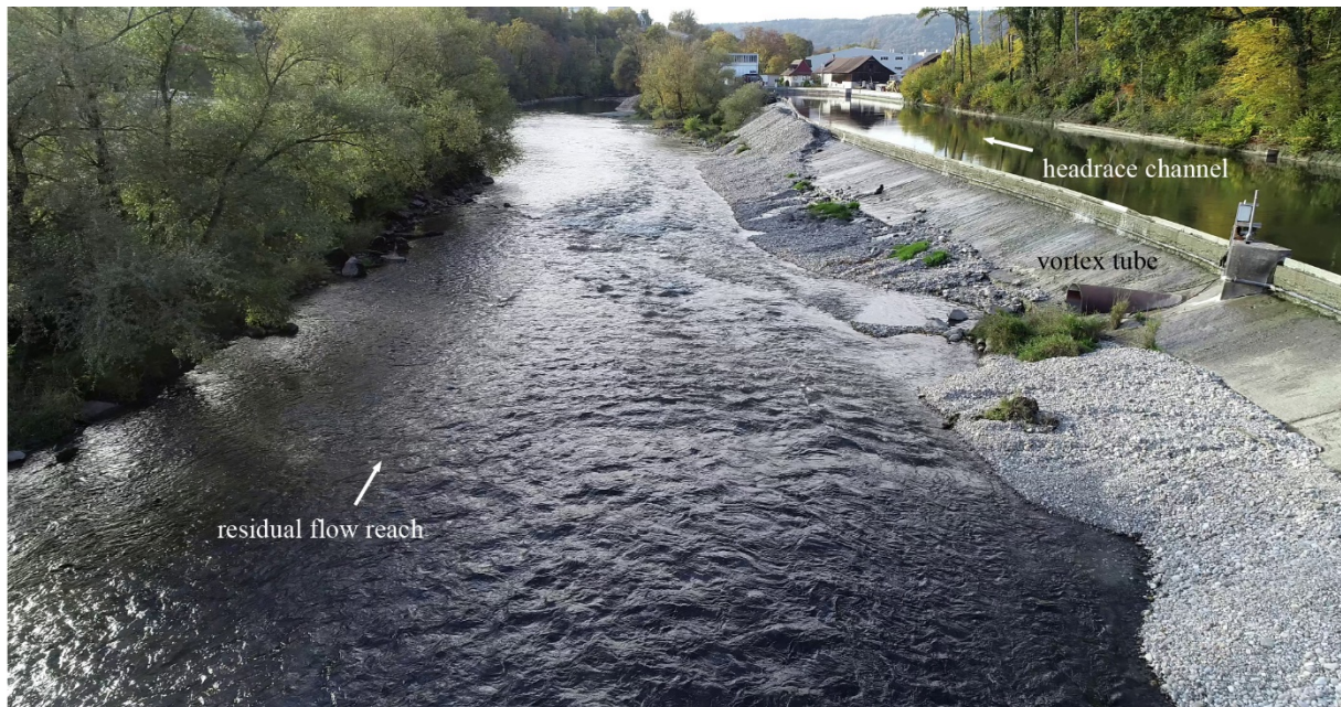
Figure 7: View of the side weir and the vortex tube at HPP Schiffmühle with the gravel extracted from the headwater channel dumped into the residual flow reach.
