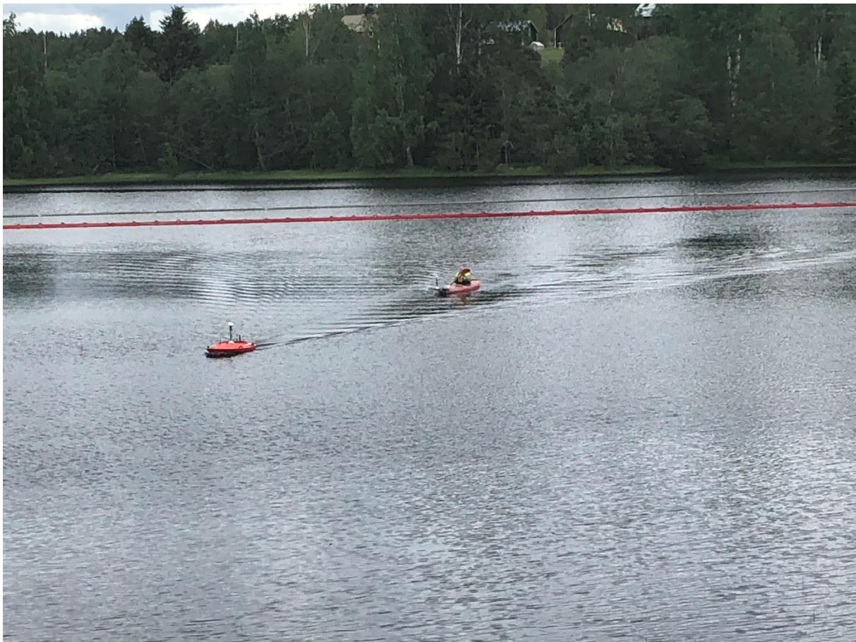
Figure 111: Barrier guiding towards the fishway entrance approx. in the middle of the lake (red line)
