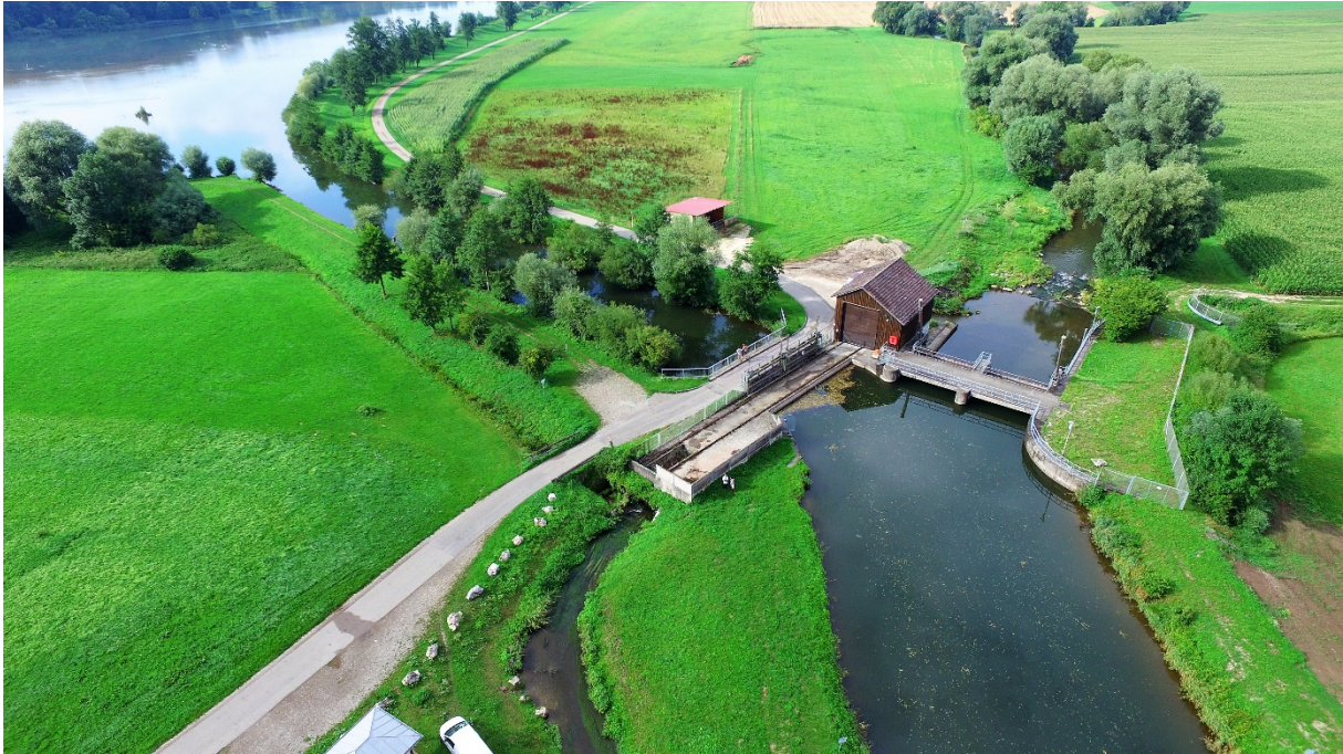
Figure 7: Teilungwehr Günz Channel and Old Günz HPP Oberegg
