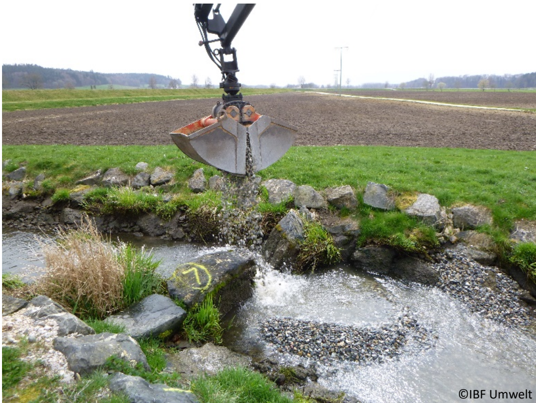
Figure 11: placing gravel into fish ladder Wattenweiler
