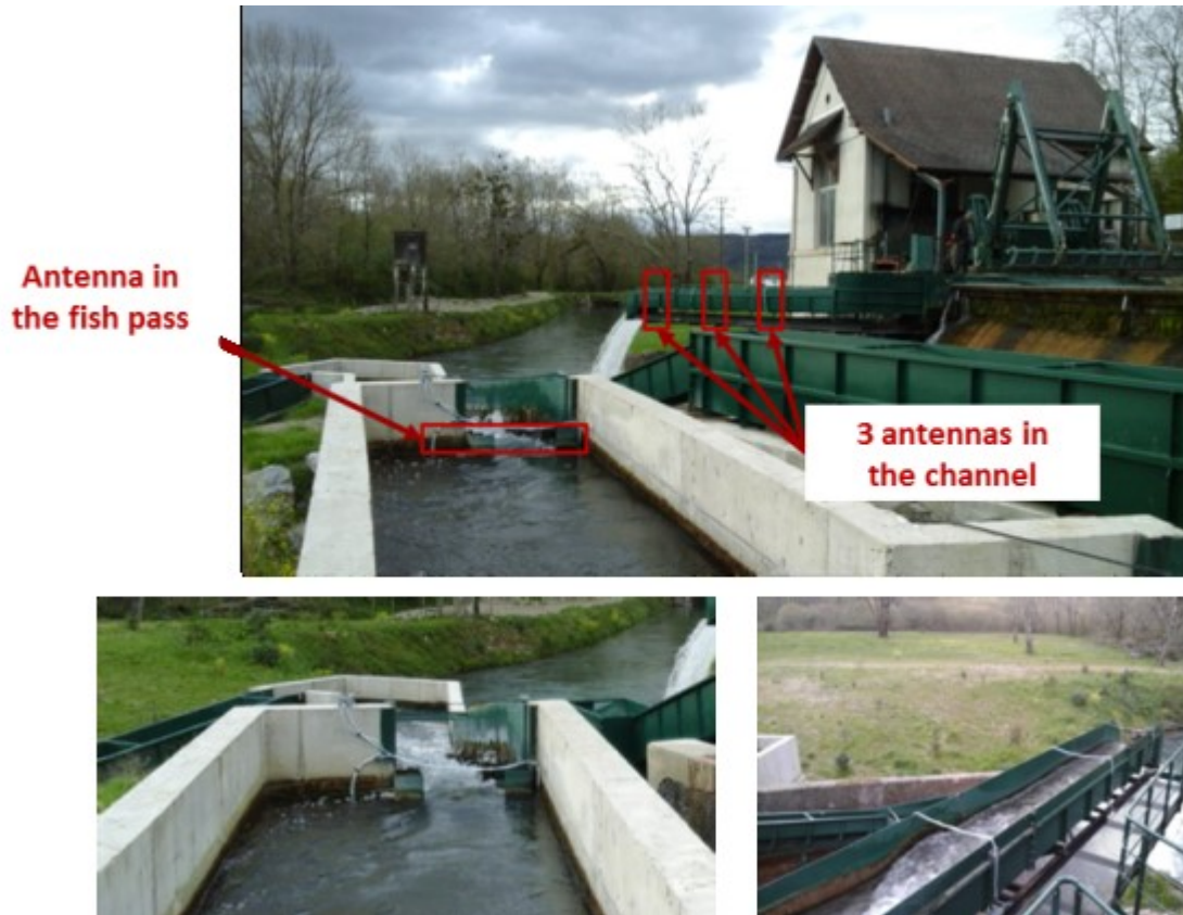
Figure 16: Pictures of the HPP and location of the antennas (source: (Tomanova, et al., 2018))
