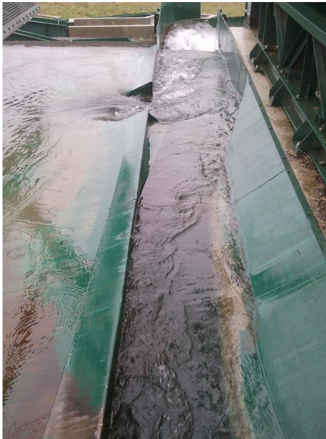
Figure 9: View of the migration duct with an enlargement at the entry of the second outlet
