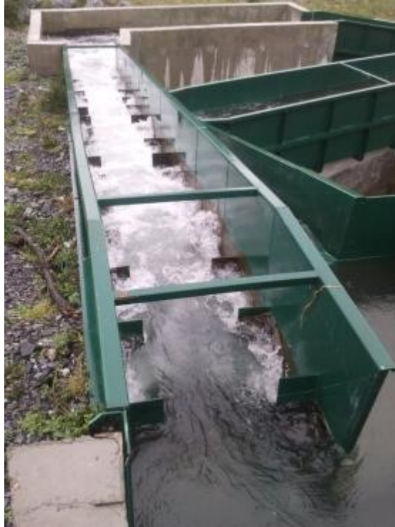
Figure 13: upstream view of the baffle fishway
