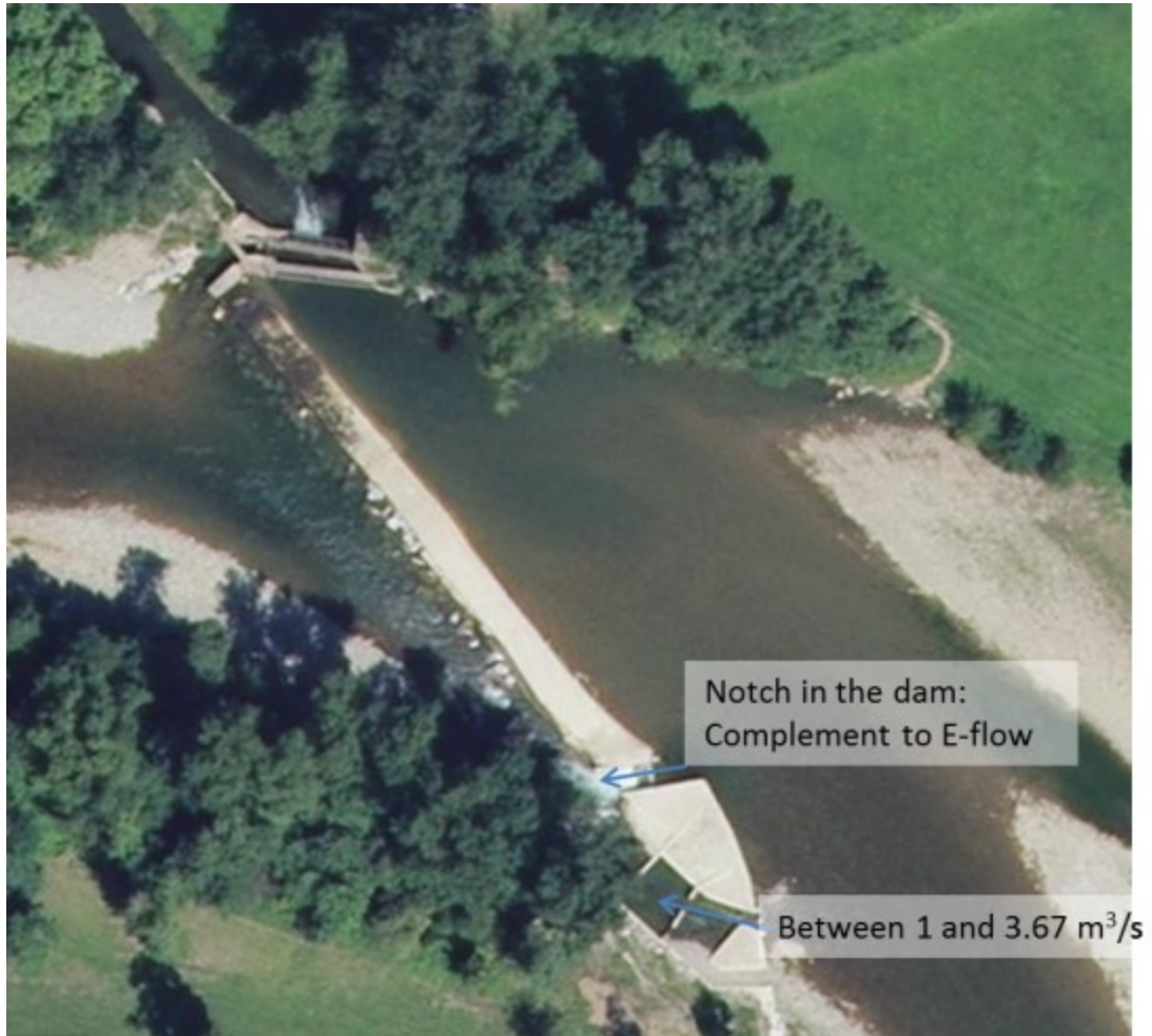
Figure 11: Location of the fish pass at the dam
