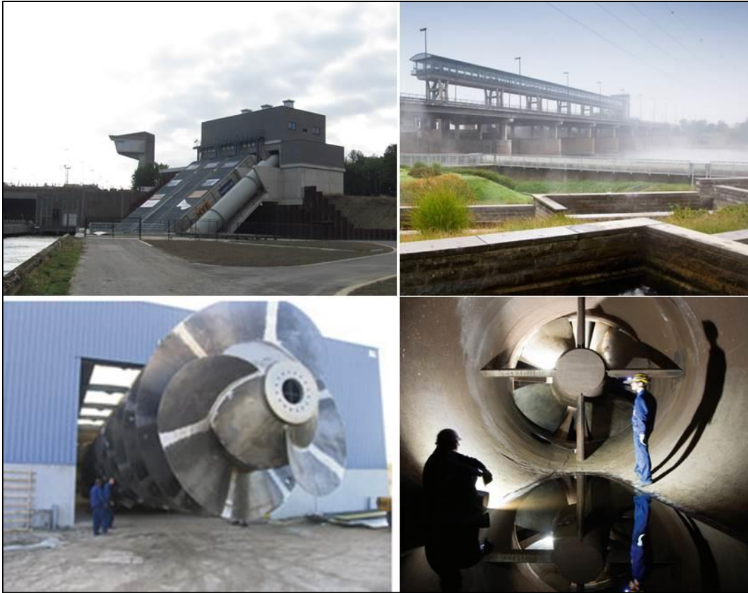
Figure 6: The pictures on the left apply on the Albert canal and visualize the pumping/hydropower station of Ham (top left), and one of the screws during its construction phase (bottom left). In contrast, the pictures on the right visualize the hydropower station of Lixhe on the Meuse river (top right) and its type of propeller (a propeller from a Straflo turbine; bottom right; sources: INBO, http://edfluminus.edf.com/ & http://www.dvo.be/ )
