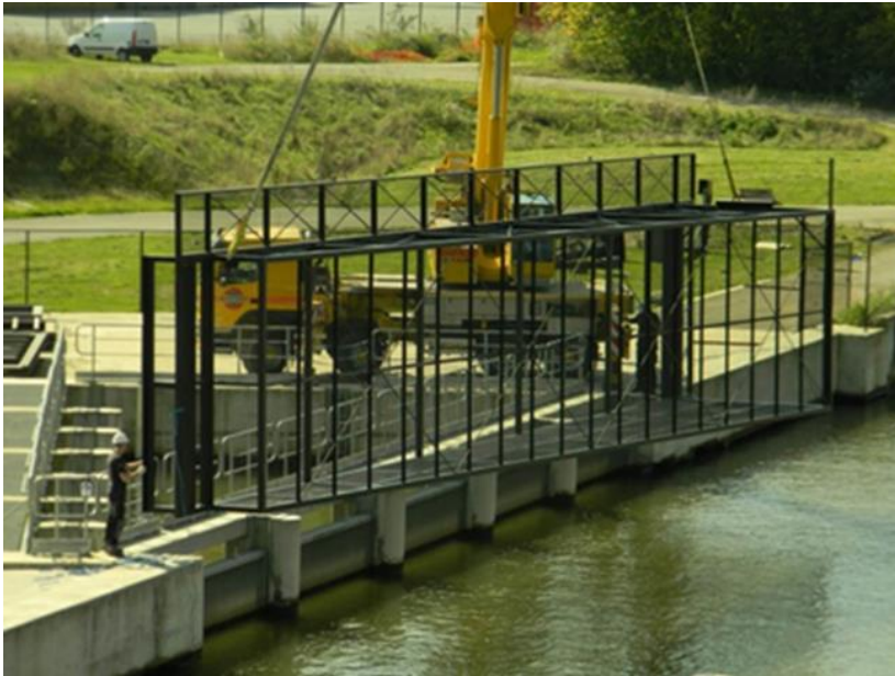
Figure 11 Picture of the installation of the cage to catch tested fish after screw passage (see also Figure 7).
