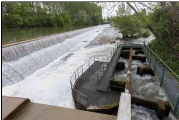
Figure 23: upstream view of the fish pass
