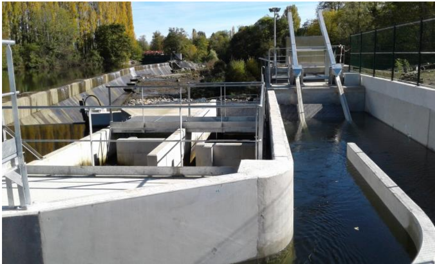
Figure 27: Fish pass and the new DIVE turbine on the bypassed reach
