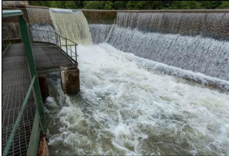
Figure 26: former notch in the weir
