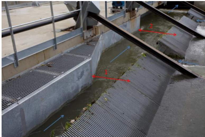
Figure 45: Positioning of the gaugings in the downstream migration duct at Las Rives
