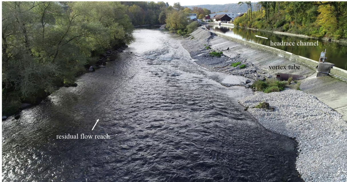
Figure 7: View of the side weir and the vortex tube at HPP Schiffmühle with the gravel extracted from the headwater channel dumped into the residual flow reach.
