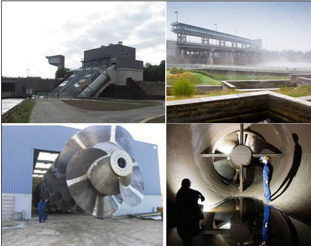
Figure 6: The pictures on the left apply on the Albert canal and visualize the pumping/hydropower station of Ham (top left), and one of the screws during its construction phase (bottom left). In contrast, the pictures on the right visualize the hydropower station of Lixhe on the Meuse river (top right) and its type of propeller (a propeller from a Straflo turbine; bottom right; sources: INBO, http://edfluminus.edf.com/ & http://www.dvo.be/ )
