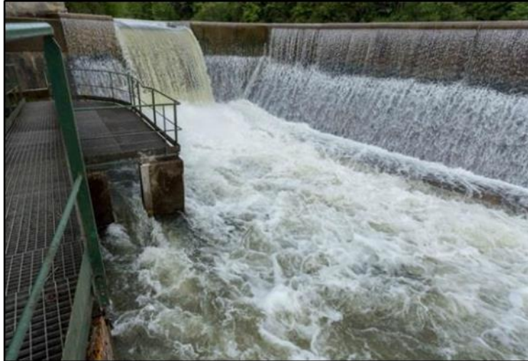
Figure 26: former notch in the weir
