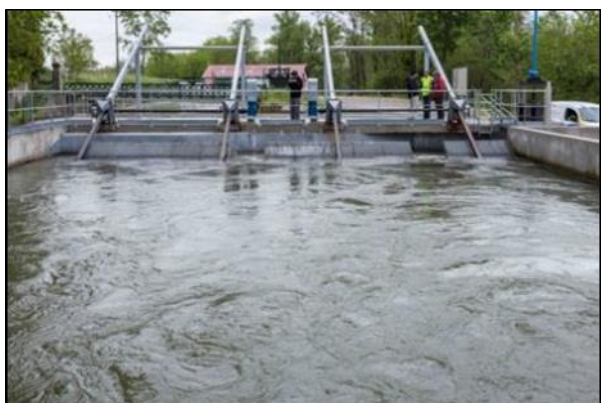
Figure 14: bar screen in water
