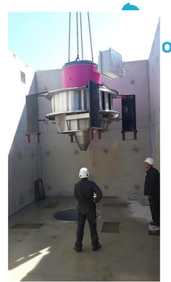
Figure 8: New Dive turbine in the headrace channel (2015) (source: www.dive-turbine.de )
