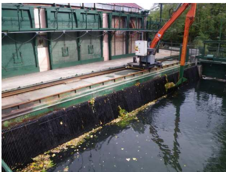
Figure 21: Bar rack in front of the HPP from 2010 to 2014 (Ecogea, 2011)
