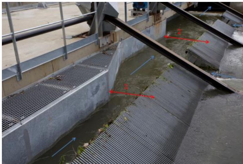
Figure 43: Positioning of the gaugings in the downstream migration duct at Las Rives
