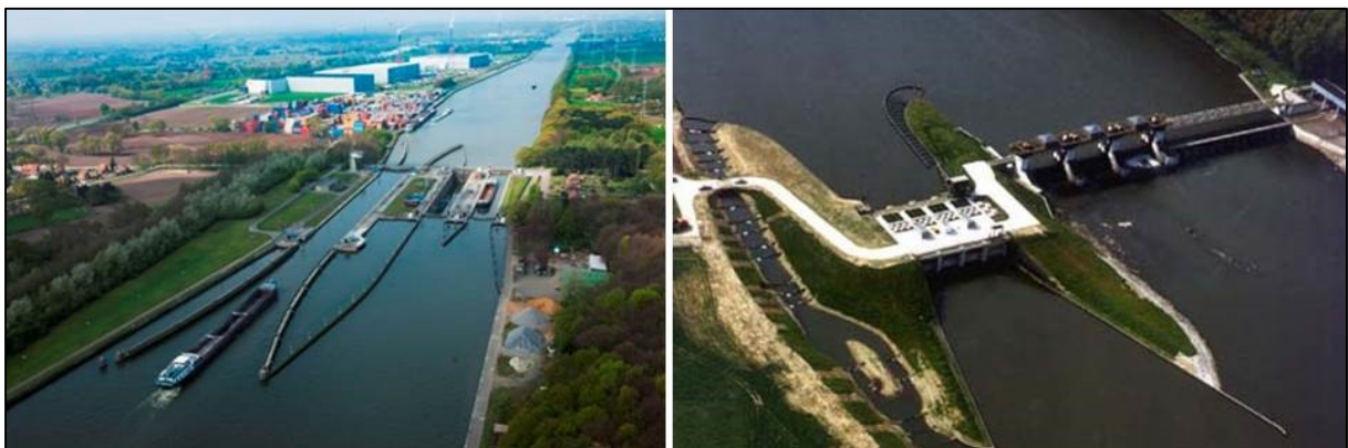
Figure 3: Lock complex in the Albert Canal (Ham) on the left and a weir complex with hydropower plant (Linne) on the right. (Source: http://nts.flaris.be/ and http://www.microhydropower.net/ )
