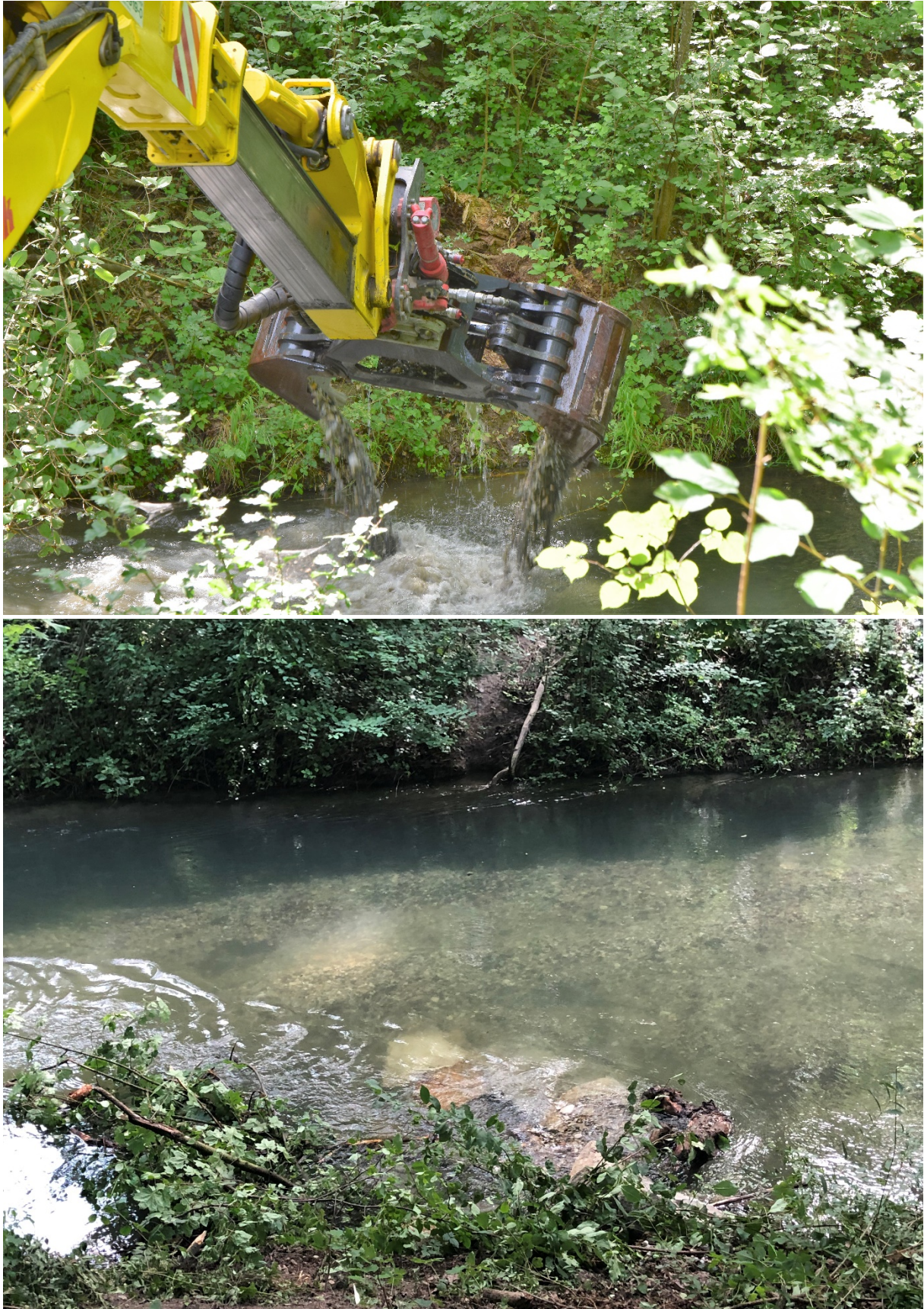
Figure 6: Structural measures for the improvement of habitat in the fishway. Top: adding of gravel; Bottom: deadwood and gravel banks
