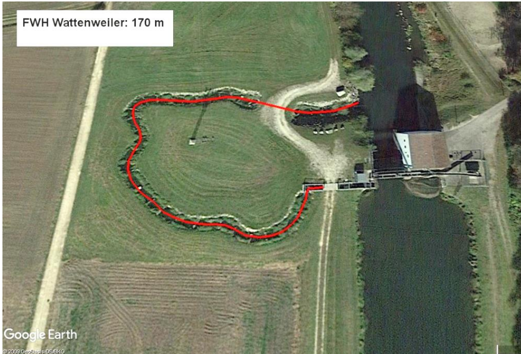
Figure 20 Aerial photo fish ladder Wattenweiler
