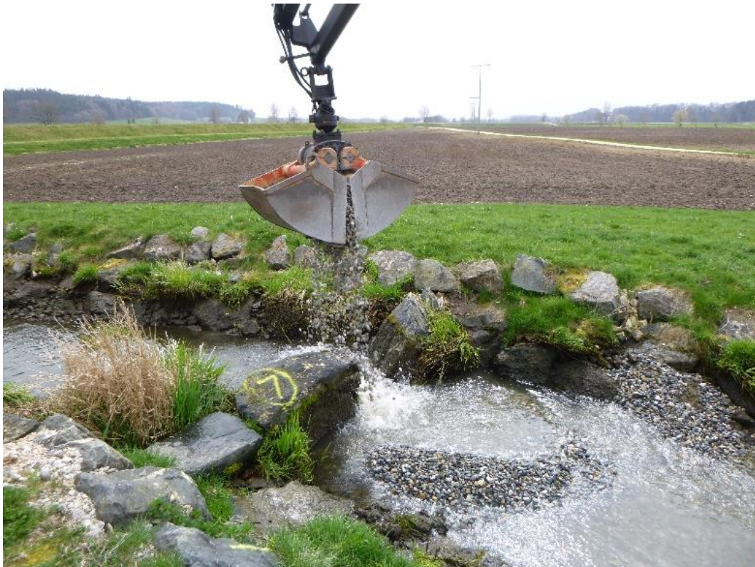
Figure 11: placing gravel into fish ladder Wattenweiler
