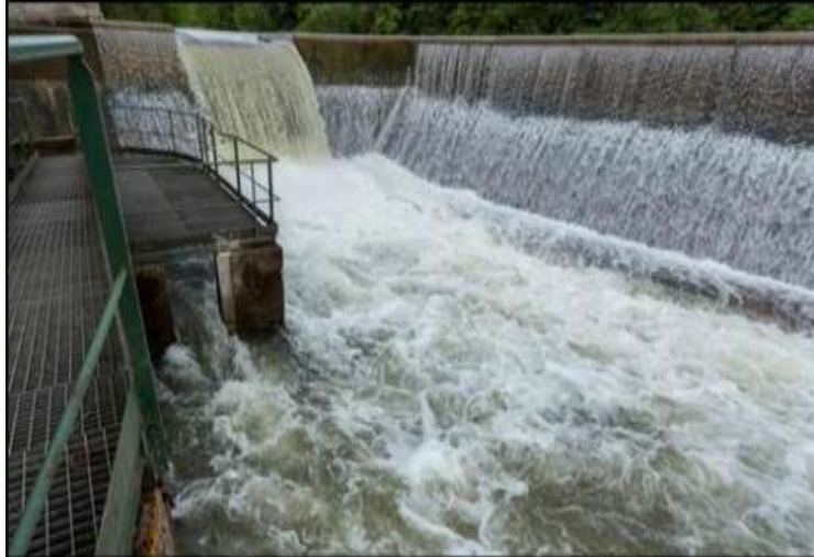
Figure 26: former notch in the weir
