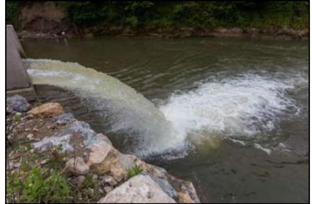
Figure 15: outlet of the downstream migration channel
