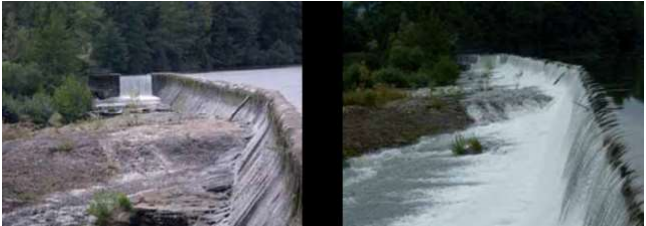
Figure 30: left pile of gravels blocking the passage of fish. Without spill, the fishes don't go in the left branch. Right picture taken when the dam is spilling (source: Rapport Ecogea, 2011)
