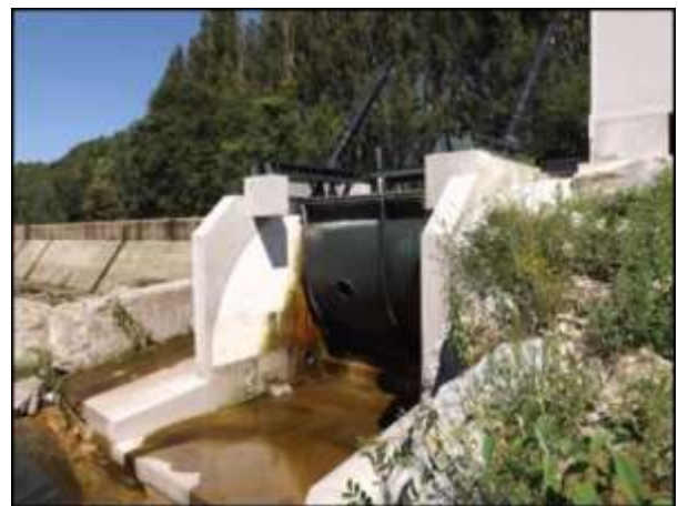
Figure 16: Dump valve for sediments
