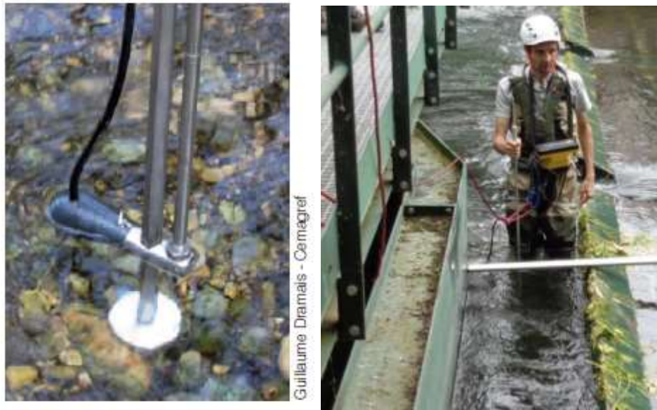
Figure 46: Example of an electro-magnetic flow meter and an operator in position in the downstream migration duct
