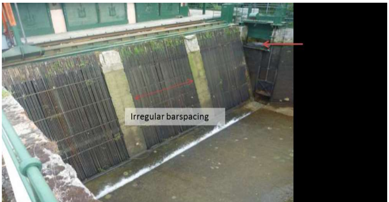
Figure 17: View of the former bar rack at the power plant (source: (Ecogea, 2011))
