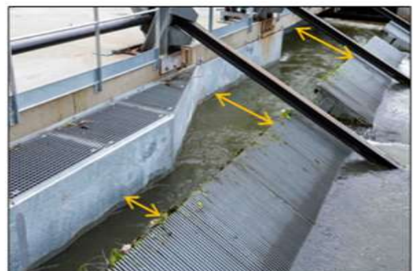
Figure 12: downstream migration duct
